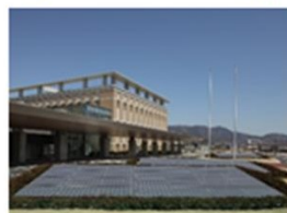
Solar energy panels
