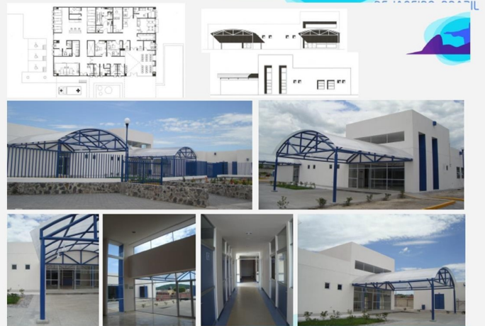
Emergency Care Center "UNEME" , Ministry of Health, Xochitipepec City
